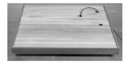
2. The bottom panel of the sauna will have the wire coming up from the floor, excluding Hybrid model (see image below)
